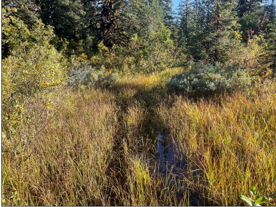
Figure 2.—Channel downstream of the culvert.
